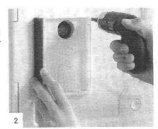
The filter casing must be installed at least 5mm from the door frame. Hold 5 mm of flats between the door frame and the filter casing as an assembly support. Insert and tighten screws, 3.5 x 16 °. VA, without pre-drilling into aluminum sheet. Apply a line of silicon caulking to the back side of the filter casing around the fan discharge opening.
