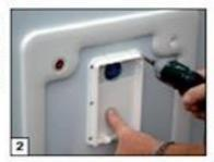
Mount the filter housing in the center of the frame recess for reasons of visual appearance. Screw screws, 3.5 x 16 mm VA, into the aluminium sheet without drilling beforehand and tighten. If a metal sheet is to be used here, pre-drill with 3 mm.
